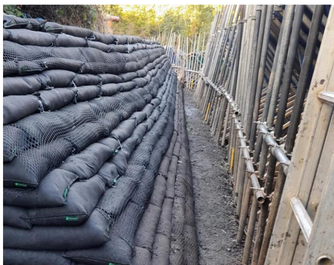
Photo 1 – Flex MSE system in place
