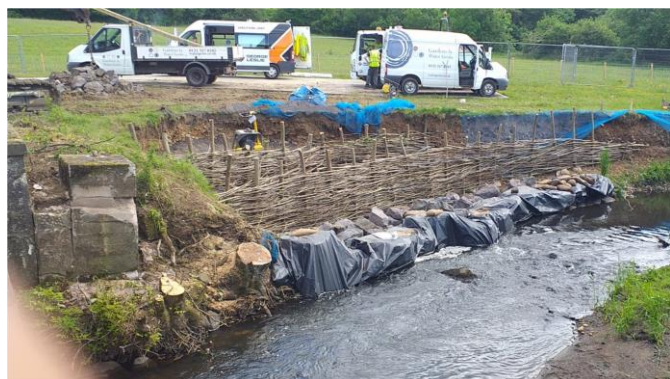
Photo 1 – install of willow along embankment
