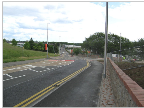
New Junction nearing completion
